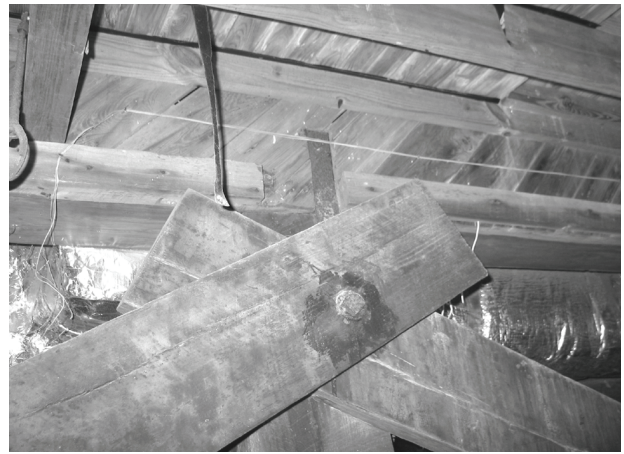
FIGURE 25. View of typical pile-beam-crossbrace
