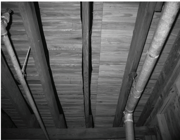
FIGURE 30. View of underside of east porch, with new flooring visible at right where older flooring has been removed. (NPS-SERO-CR, 2003)
