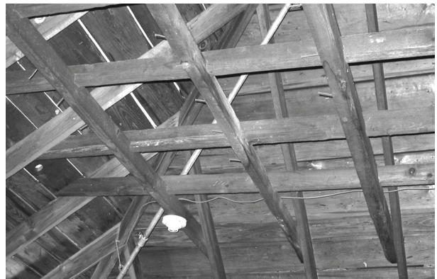
FIGURE 32. View northwest in attic showing cross-braced collar beams on main roof. (NPS-SERO-CR, 2003)
