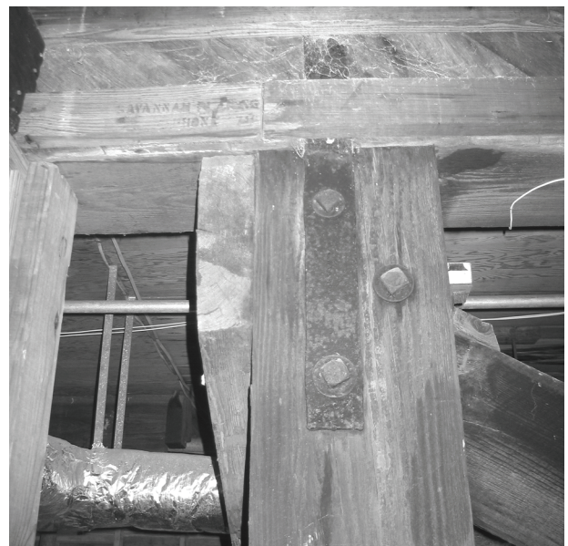
FIGURE 26. View of typical iron strap that secures house framing to pilings. (NPS-SERO-CR, 2003)
