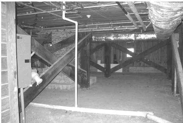
FIGURE 24. View west under north porch, showing typical piles and cross-bracing. (NPS-SERO-CR, 2003)
