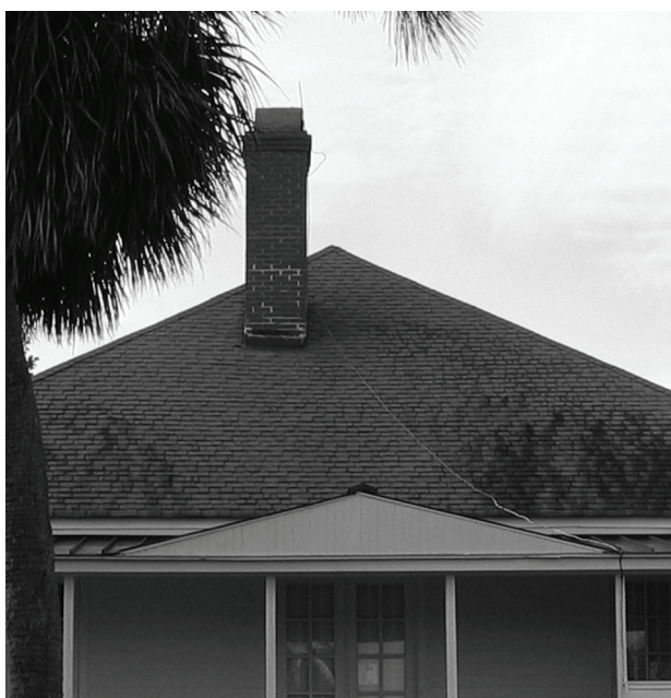
FIGURE 35. View south, showing modern gable over porch entrance. Note that modern fascia replaces original crown molding. (NPS-SERO-CR, 2003)
