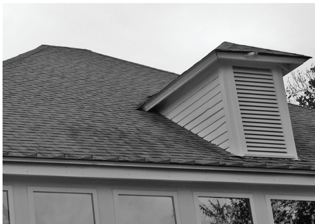
FIGURE 34. View east, showing original dormer. Note that modern fascia replaces original crown molding. (NPS-SERO-CR, 2003)
