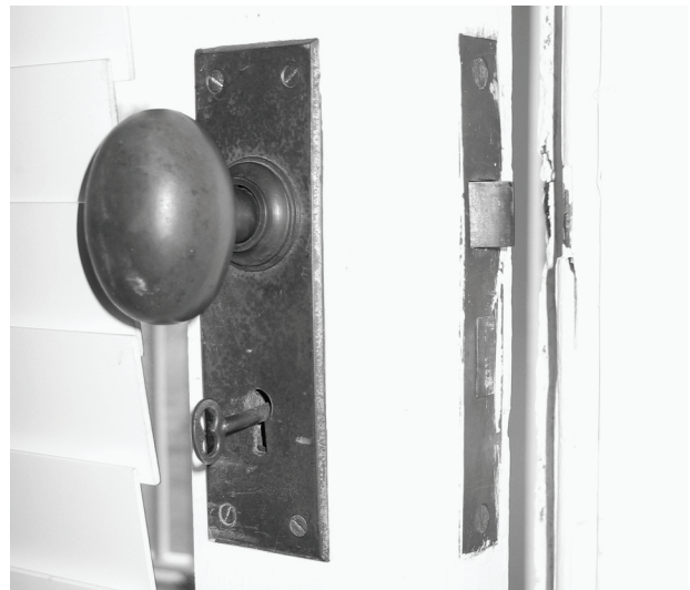
FIGURE 37. View of typical mortised lock installed with French doors in 1942. (NPS-SERO-CR, 2003)
