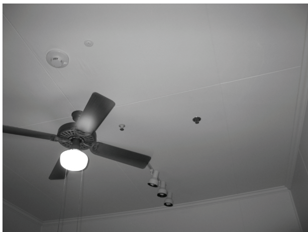
FIGURE 44. View of typical plywood ceiling installed in 1942. Beveled edges are distinctive features of this material. Similar material was used on some walls as well. (NPS-SERO-CR, 2003)
